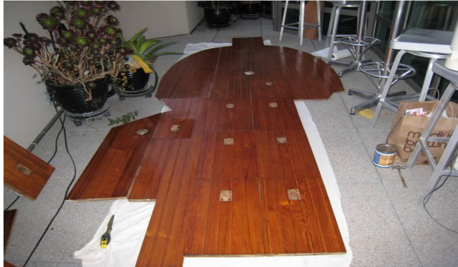
The teak sole is looking good after Bob has stripped, sanded, and sealed it. Here he has the first two coats of varnish (Ultimate Sole).
